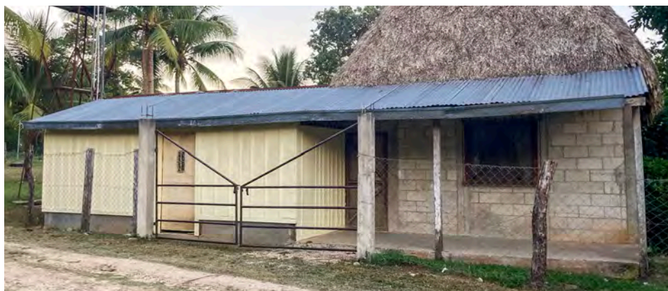
The small house in Santa Rosita before remodeling.
