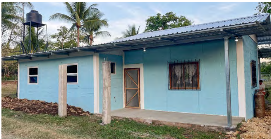
After a new roof was installed.
