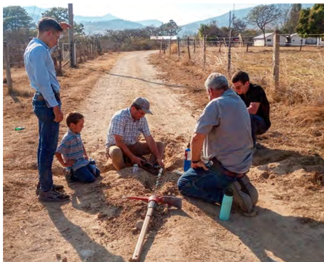
Fixing a broken water line.
