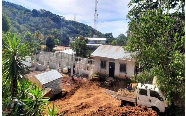
Hard-won progress on the school construction.
